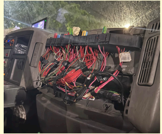
Truck with exposed electrical wires, MIA 2/10/26
